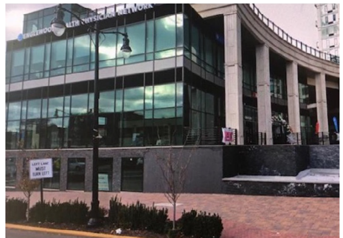
695 Anderson Ave - View from Anderson Ave facing southwest
