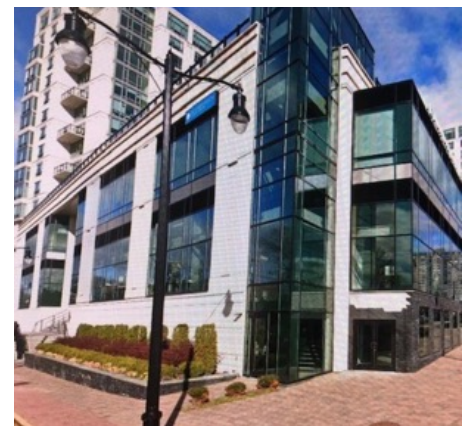
695 Anderson Ave - View from intersection of Anderson Ave and Lawson Ave
